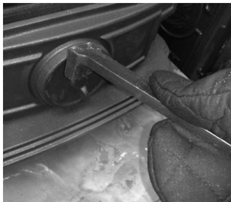
The Primary air the base of the stove door is opened, using the tool, by turning anti-clockwise
