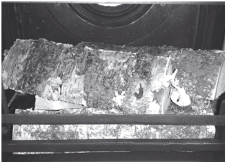
The recommended maximum fuel load: Photo shows a typical loosely stacked fuel load
