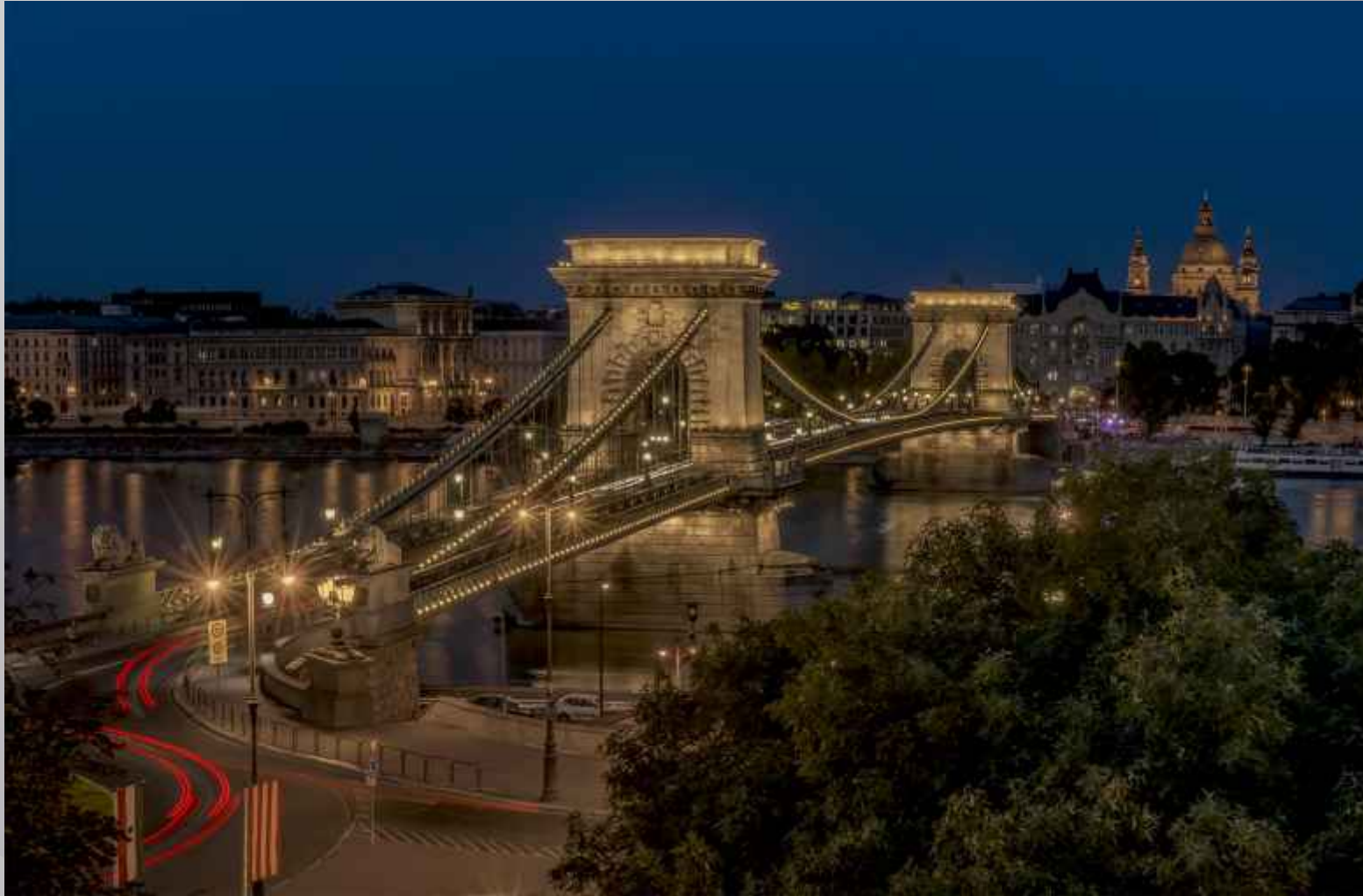
Budapest Chain Bridge
